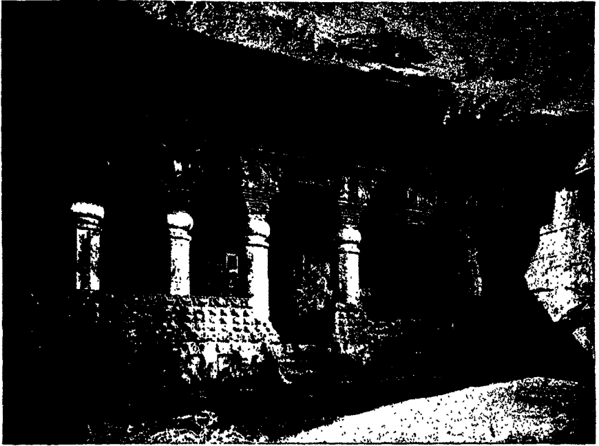
FIG. 52— Façade of the Gautami-Putra Monastery at Nasik India Office, London
